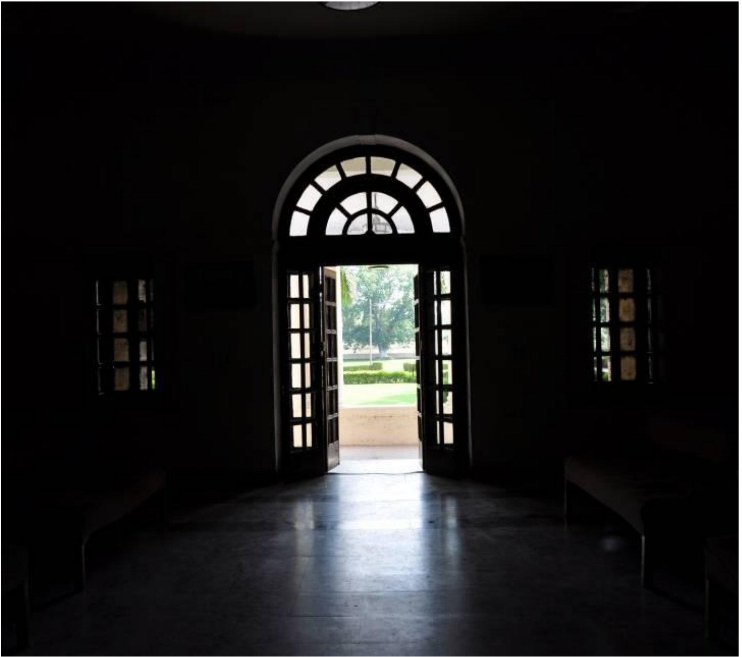
Entrance Door to Junior School, view from within
