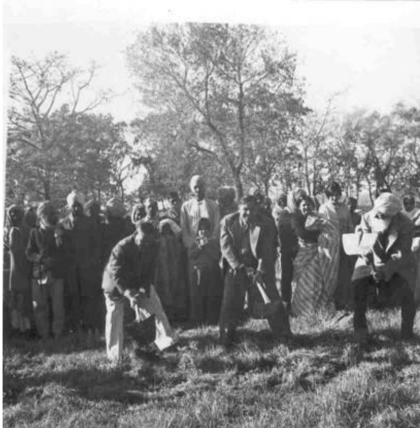
Digging for a Swimming pool, one of the innumerable structures that he added to PPS infrastructure
